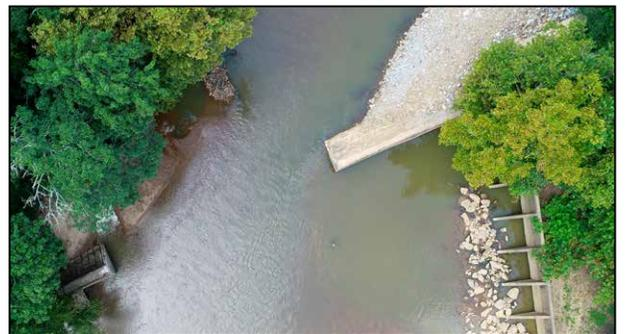
*Top: Heavy equipment operators work to remove portions of the White Dam on the Middle Oconee River. Above: Aerial photographs show the dam before and after partial removal. The project creates 22 miles of free-flowing river between upstream and downstream impoundments. The removal is expected to improve habitat for Altamaha and Ocmulgee shiners, fish that are found in the Altamaha River basin and nowhere else on Earth.*
