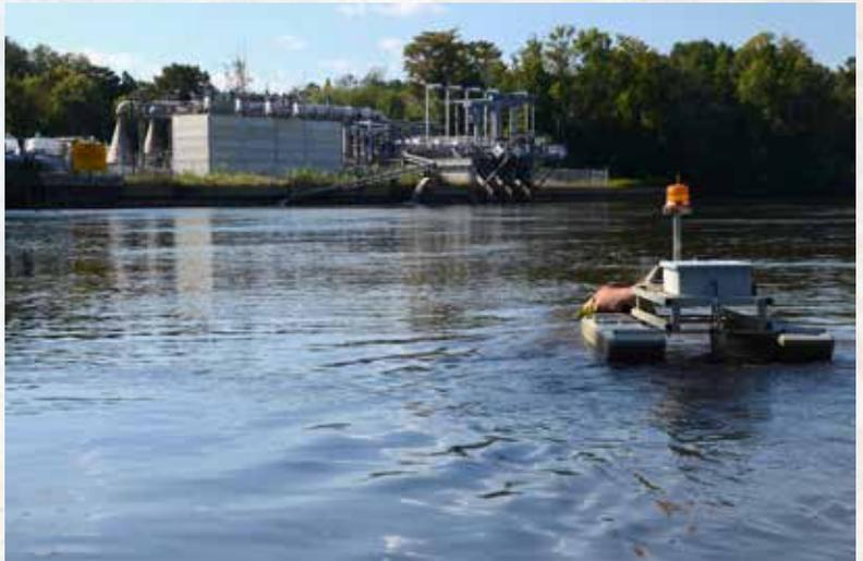
The U.S. Army Corps of Engineers dissolved oxygen injection system operates on the banks of the Savannah River. The facility injects oxygen into the river to support habitat for aquatic wildlife, including federally protected fish species. The Savannah River TMDL for dissolved oxygen forced more than 20 municipal and industrial dischargers to work to reduce their impact on the river and prompted the construction of this facility to mitigate impacts from the deepening of the Savannah Harbor.
