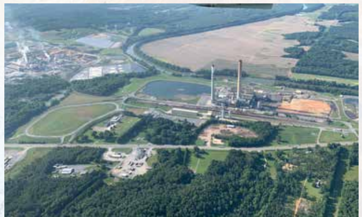
Located in the far left of this photo, Ash Pond 3 now appears as a 25-acre grassy mound along Ga. 20 in the foreground. It looms over Pisgah Baptist Church to the west and Cabin Creek to the east. It appears benign, but in fact, beneath the surface coal ash extends some 44-feet deep and ten feet below the upper limit of the groundwater table.
